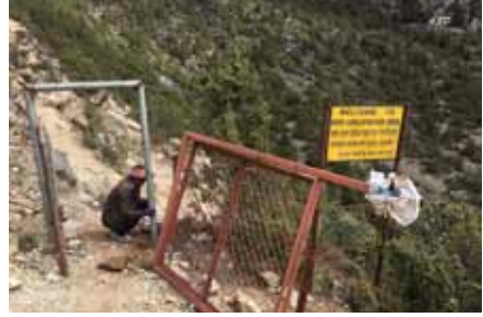
Bird conservation zone fencing and gate repair
