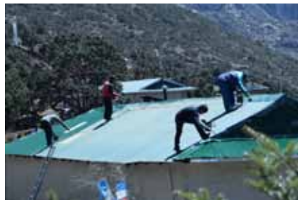
Green roof repainting
