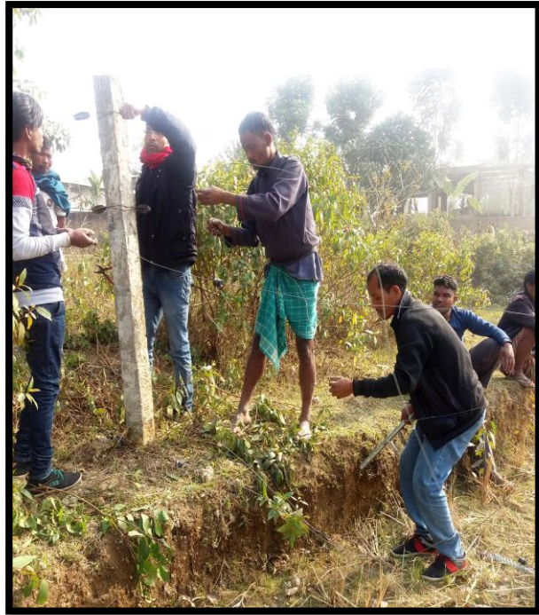
Fig. 11 Community based maintenance of solar electric fences at Kalyanpur village, Goalpara in Assam Hathi Project
