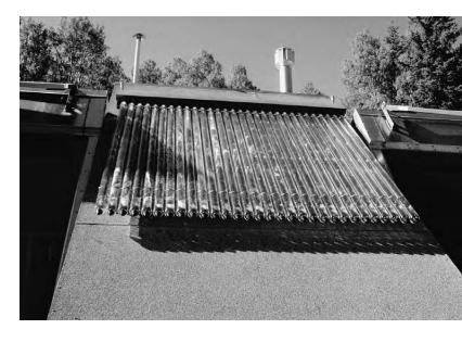
8.12: One of the newest and most efficient solar hot-water systems made by Thermomax,
