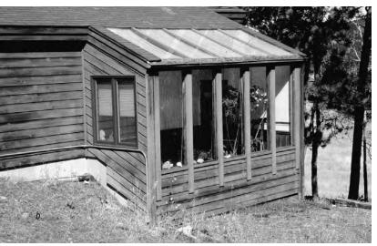
8.11 a & b: Passive solar can be added to existing homes either (a) by installing additional windows on south-facing walls or (b) by adding solar greenhouses. Credit: Dan Chiras.
