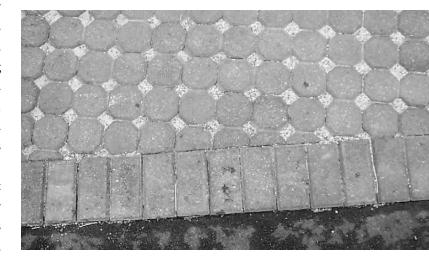
6.3: Porous pavers like these let moisture seep into the ground, reducing surface runoff, flooding, and nonpoint source water pollution. Porous pavers and other similar strategies reduce heat-absorbing pavement, making homes much cooler in the summer while reducing utility bills. Credit: Turfstone Company.
