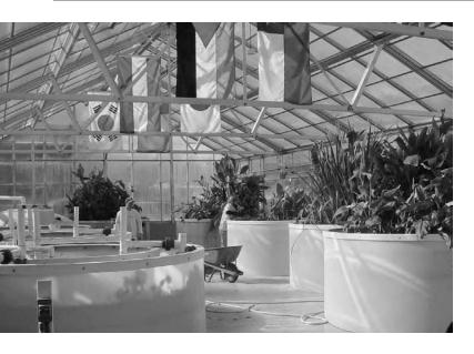
9.2: The Living Machine is a greenhouse-contained biological waste treatment facility that uses natural methods rather than harmful chemicals to recycle human waste. Credit: Stacey Giordano.
